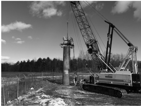
Vibratory Hammer Make sure hammer has two clamps One is for sheet pile installation!
