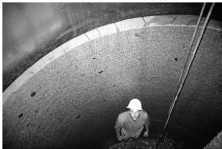
14 foot Diameter Shaft in Very Hard Granodiorite!
