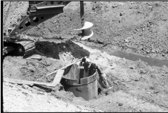
Remember, even a temporary loss of focus can be dangerous
