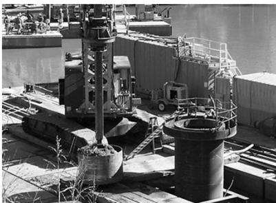
Cleanout bucket in operation
