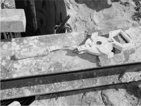
Check Depths with a Weighted Tape
