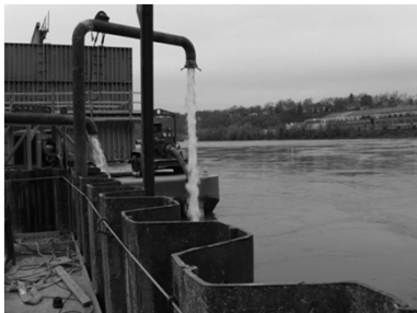
Lots of water when 60 feet below the river!
