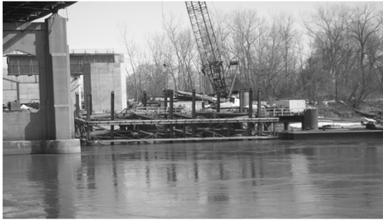
Atchison River Coffer Dam Drop
