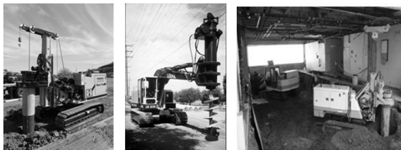
The Lo-Drill , a low-clearance rig
