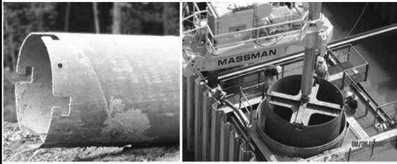
“twister” fits into slots in casing, allowing drill rig to apply torque and crowd
