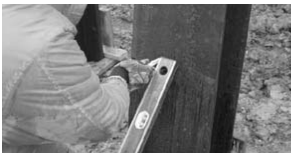
Figure 7 Mark pile as Driving Continues
