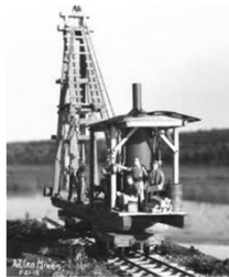
Rail Road Steam Pile Driver 1912
