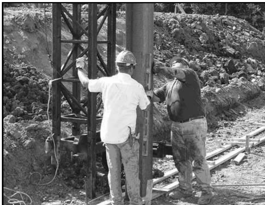
Figure 5 Plumbing an H-Pile
