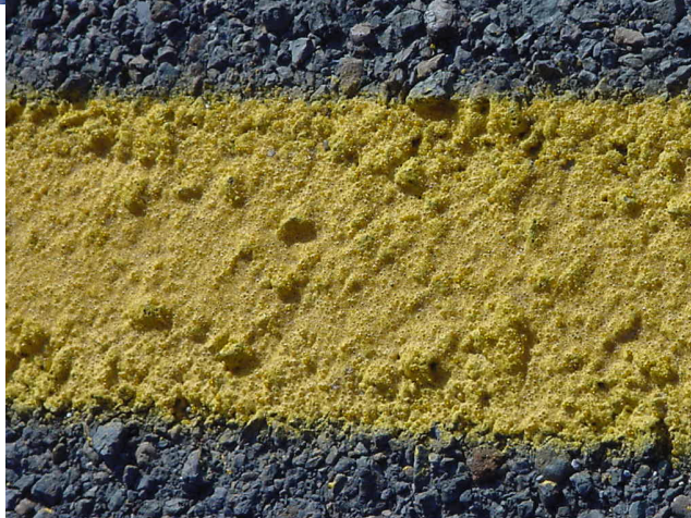
Yellow paint with glass beads on rocky asphalt surface.
