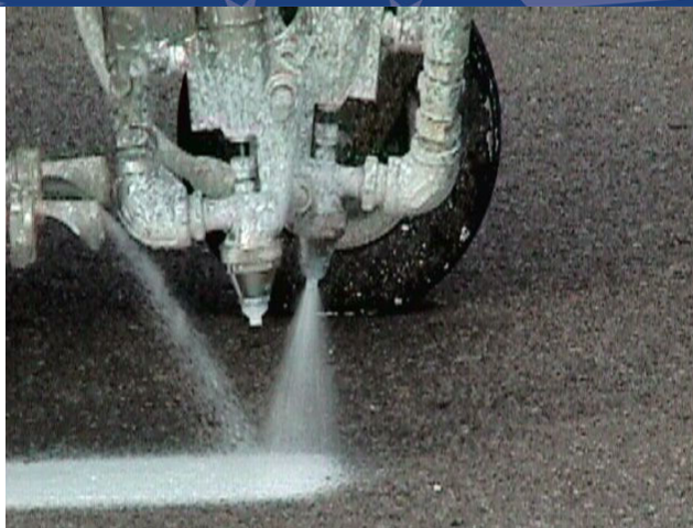
Paint being sprayed on road and glass beads dropping on the sprayed paint.
