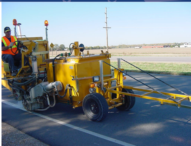
White thermoplastic being applied to road surface.
