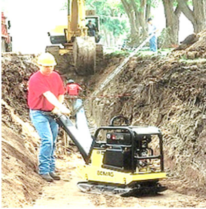
Vibratory Plate Compactor (Wacky Packer)
