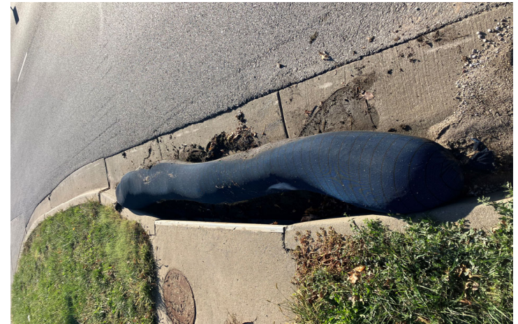
CURB INLET PROTECTION
