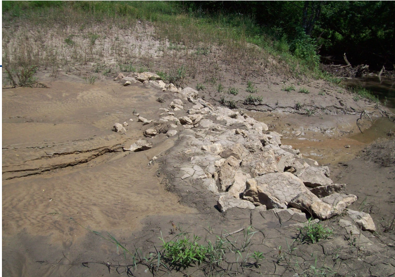
This shows an effective rock check. The sediment does need to be removed from behind the check.
