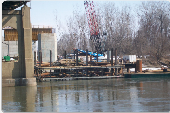
Atchison River Cofferdam Drop
