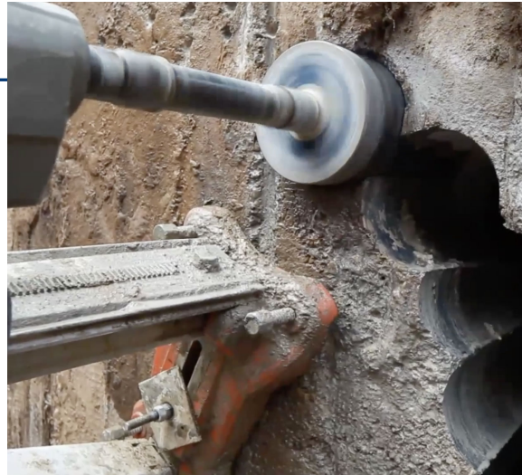
Coring in-situ concrete
