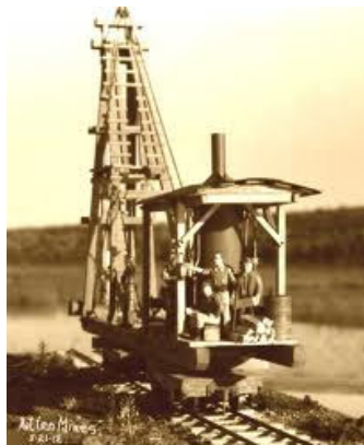
Railroad Steam Pile Driver 1912
