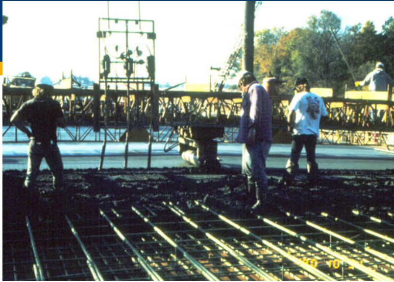
(Mud placement, Single Drum Screed, Gang Vibrators) (CHECK/RECORD Cover & Fillet Depths at 10 th Points)
