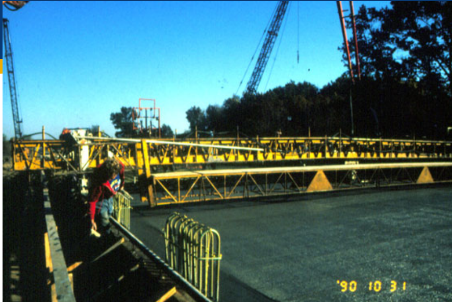
Float Train c. '90 (Transverse Grooving now done by multi-blade diamond arbor, see Sub-Sec. f., p. 700-46)
