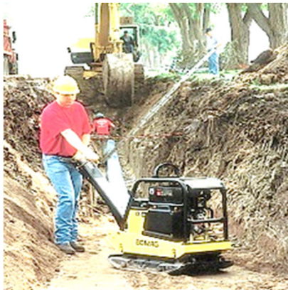
Vibratory Plate Compactor (Wacky Packer)
