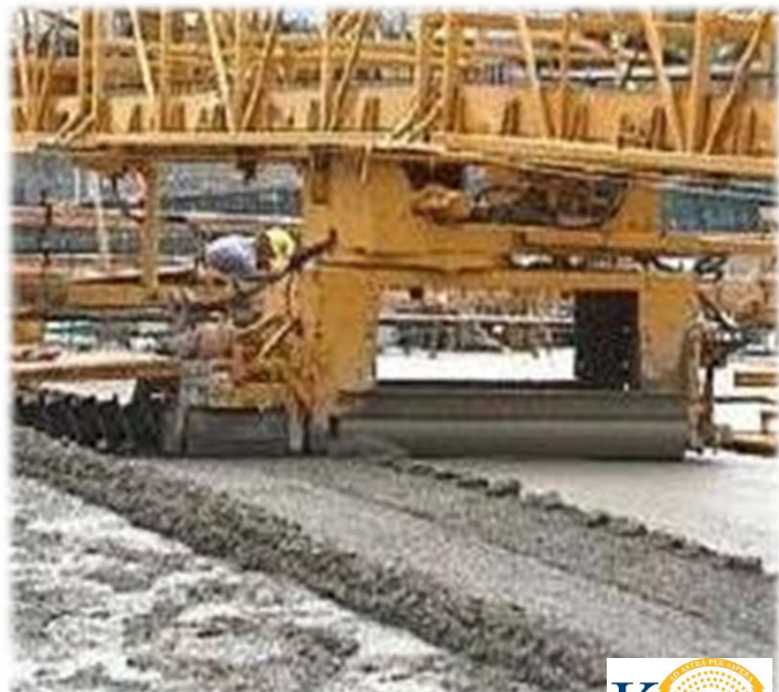
Traveling Carriage Screed (Up-Close)
