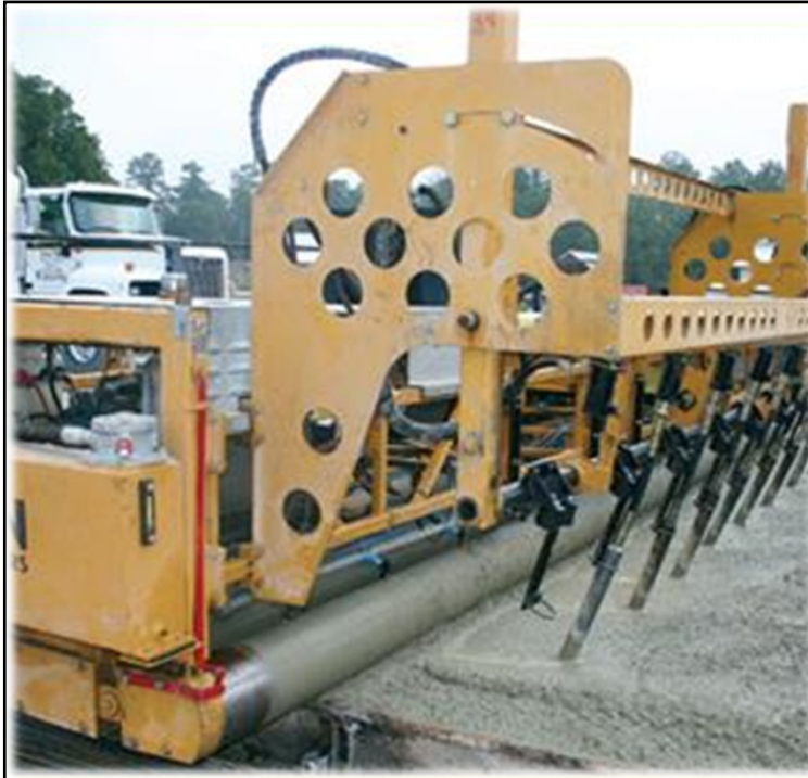
Self Propelled Roller Screed
