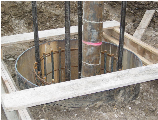
Mark tremie/ discharge tube
