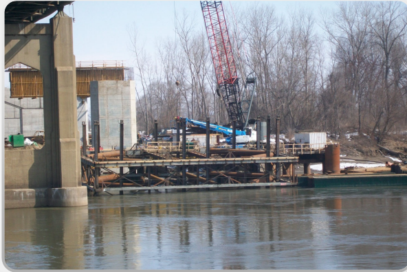
Atchison River Cofferdam Drop
