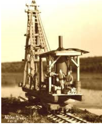
Rail Road Steam Pile Driver 1912
