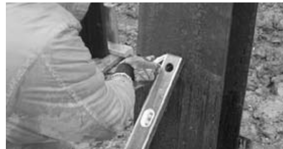
Figure 10 Continue Driving Until Bearing
