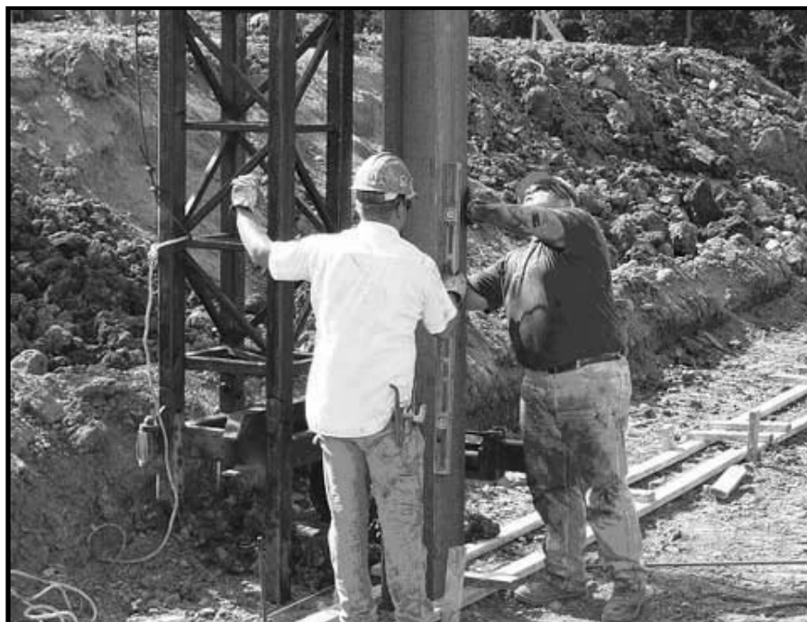
Figure 5 Plumbing an H-Pile
