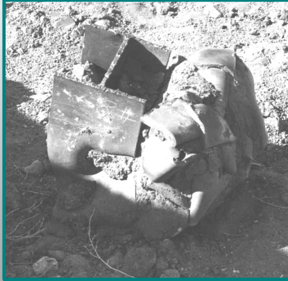
The lower 7 feet of Pile #5 at Pier 1.
